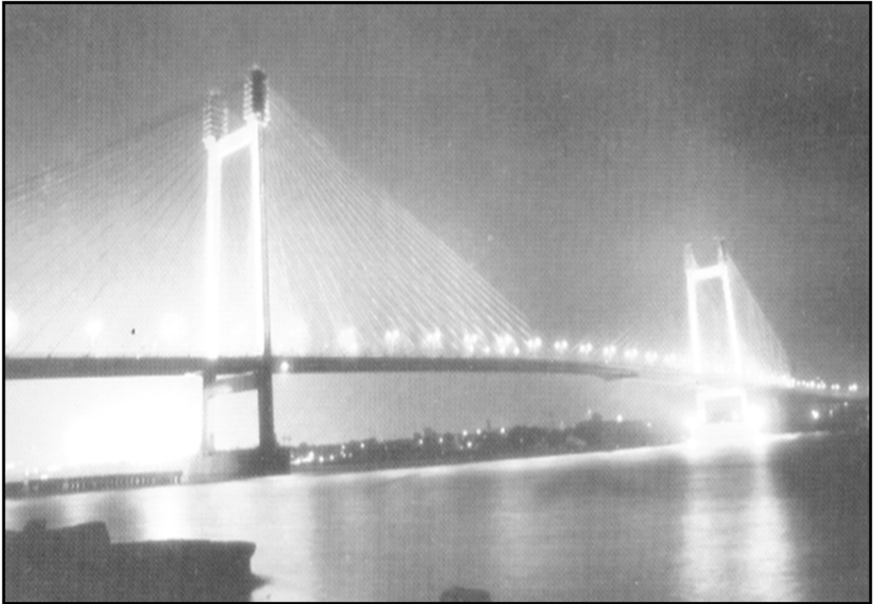
The second Hooghly cable stayed bridge 1992
