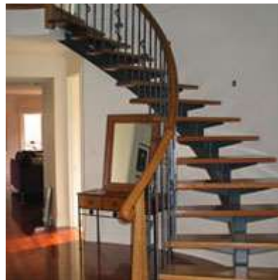
Transversely spanning SC
