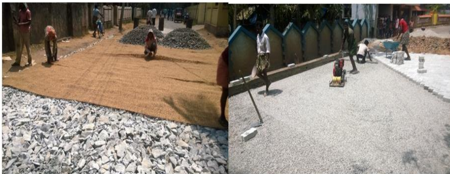
Construction of ICBP at Channankara using Coir Geo Textile
