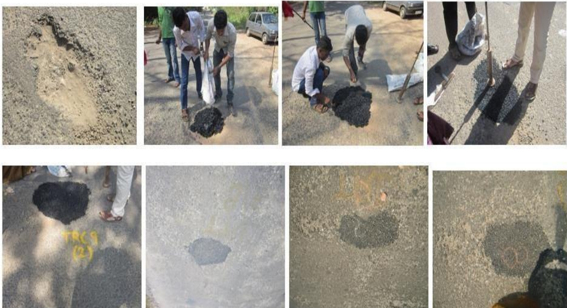
Fig.8 Trial filling of potholes on Kariavattom – Thrippadapuram road
