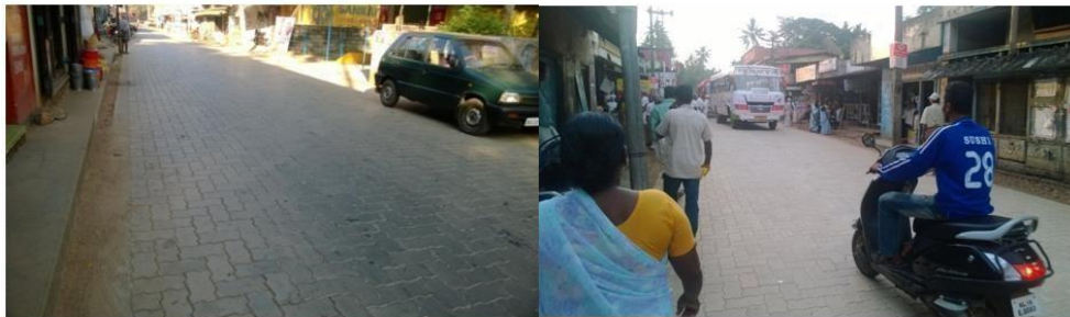
Condition after the construction using Interlocking concrete Blocks at Vakkom Market Jn.
