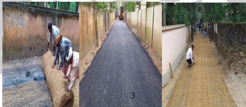
Fig.2 Overlay of coir geotextiles
