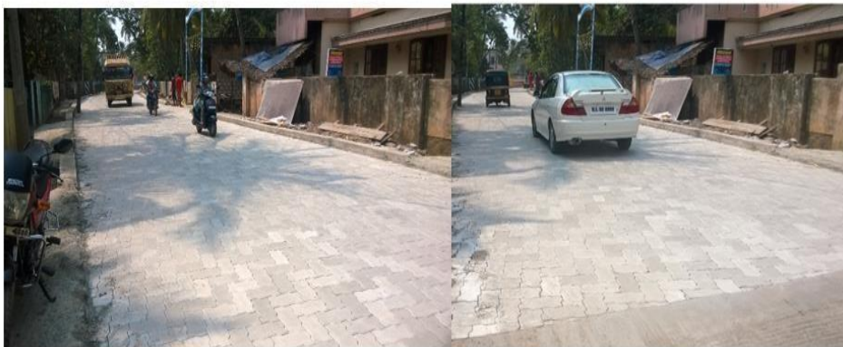
Condition after the construction using Interlocking concrete Blocks at channankara
