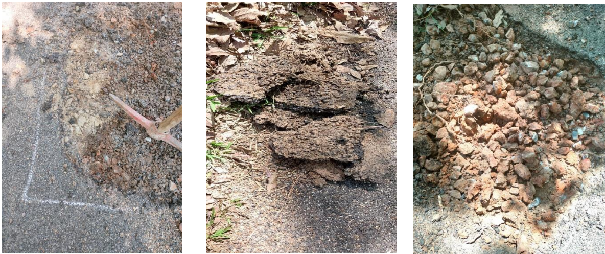
Fig 8: Separately collect various pavement layers
