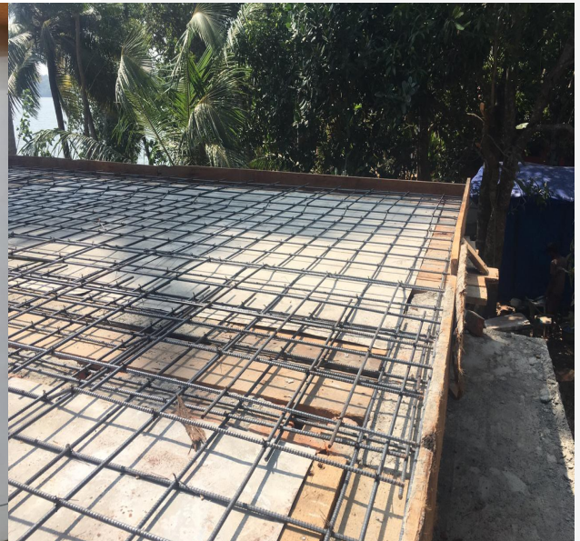
Layout of the reinforcement used
