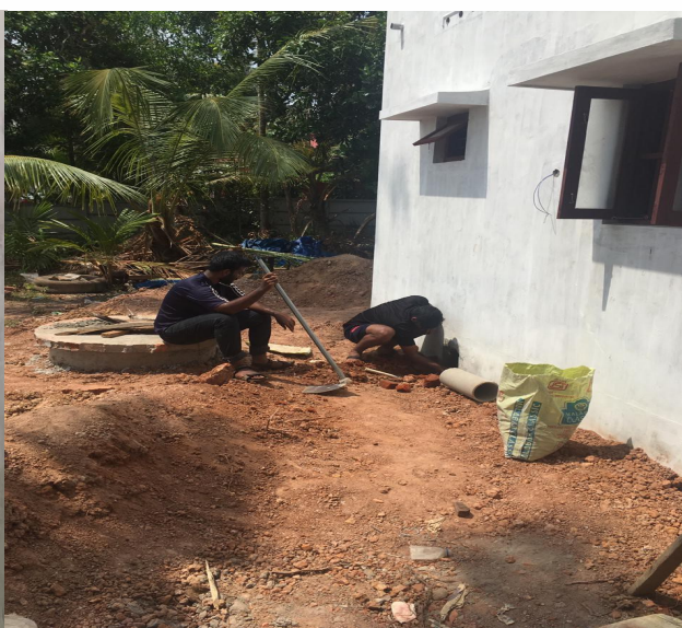
Students digging out a ridge to allow drainage flow
