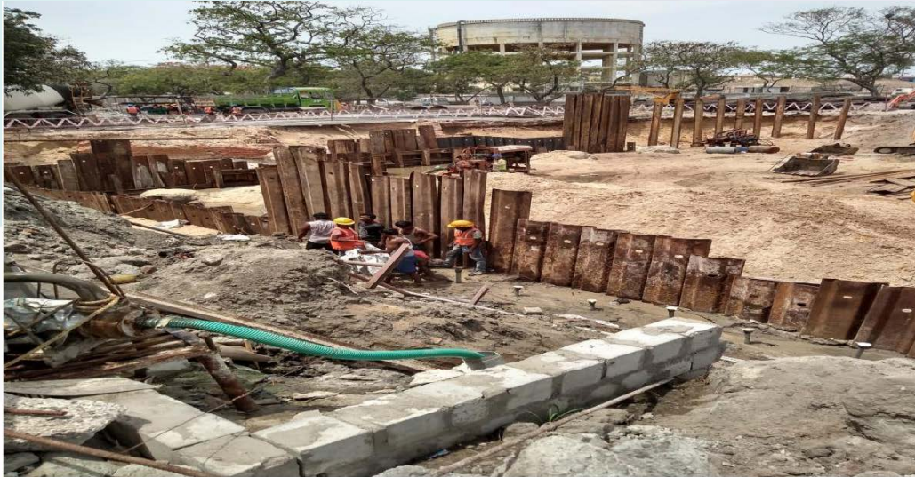
Construction of UG tank
