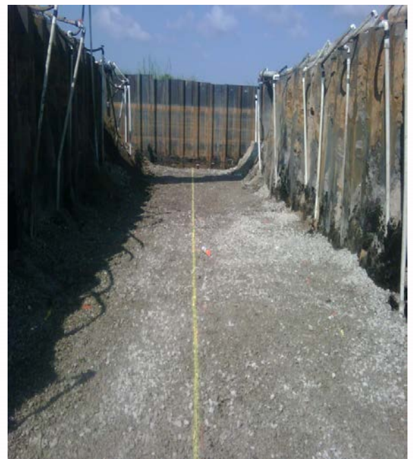
Construction of dewatering well
